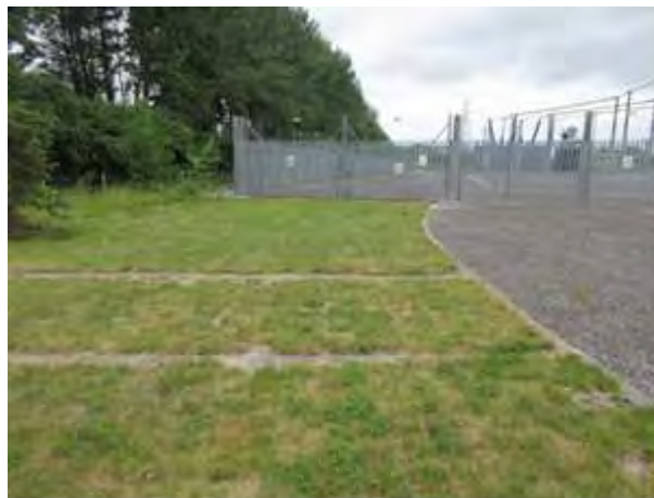
Reference Image 2 Example of a substation access road constructed of Grasscrete.
