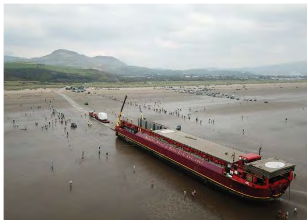
Reference Image 4 Example of an access road constructed using trackway across beach to enable beach landing of AIL.
