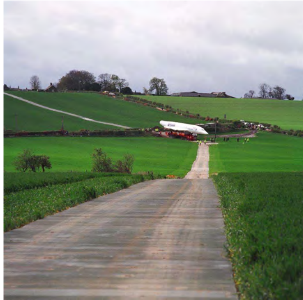
Reference Image 3 Example of an access road constructed using trackway across fields.
