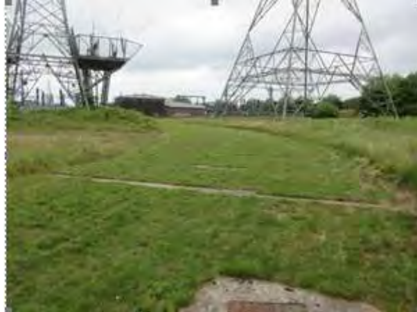
Reference Image 1 Example of a substation access road constructed of Grasscrete.
